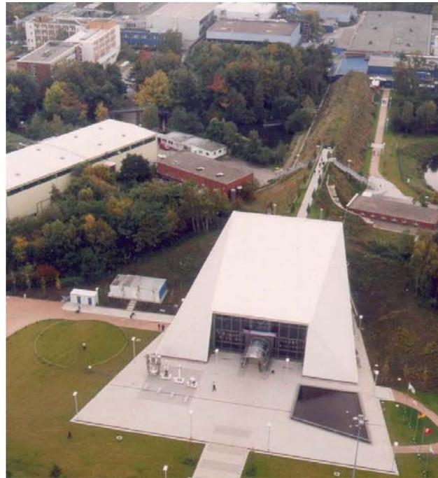
Figure S1: Aerial view of the experimental hall for the FLASH User Facility in Hamburg (center) and the tunnel for the superconducting accelerator and undulator (covered with grass). The hall in the upper right corner houses the injector section of the linac. The total length of the FLASH facility is 300 meters. The maximum energy of electrons is 1 GeV, and the minimum radiation wavelength is 6 nm.
