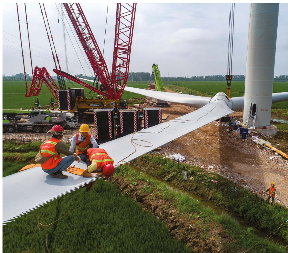
Wind turbine blades are secured and examined before being hoisted into position in China's Jiangsu province.
