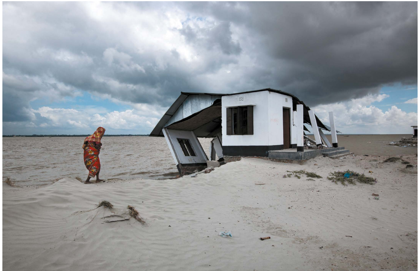
A damaged temporary home near the Meghna River in Bangladesh, in a coastal area threatened by erosion and rising saltwater levels in soil.
