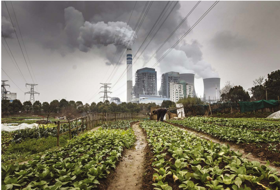
A coal-fired power station in Tongling, China.
