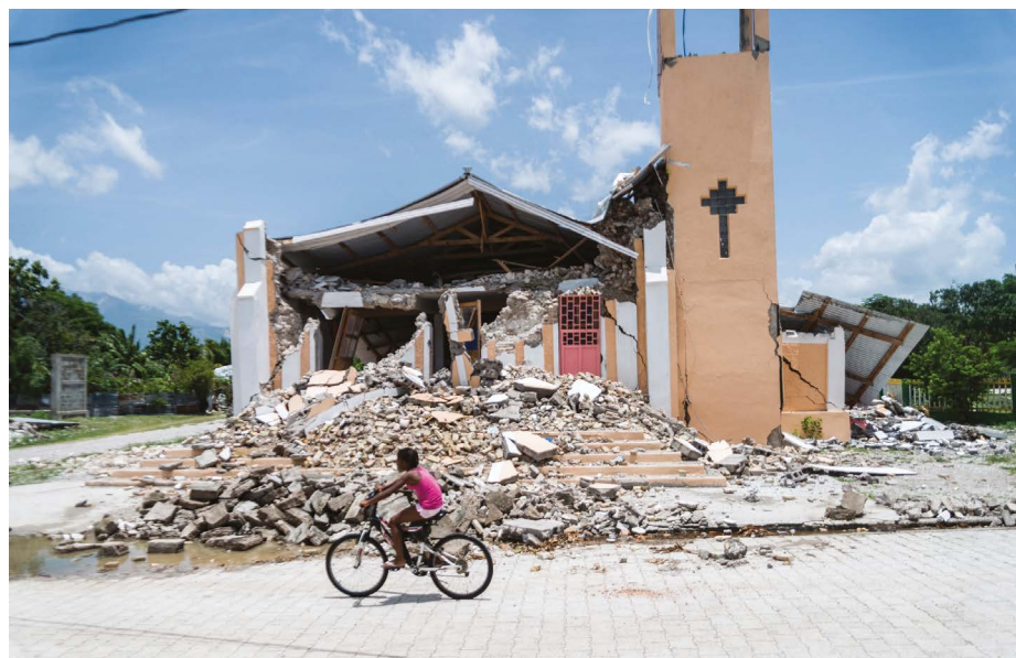
Haiti's earthquake last month destroyed many buildings, including this church.
