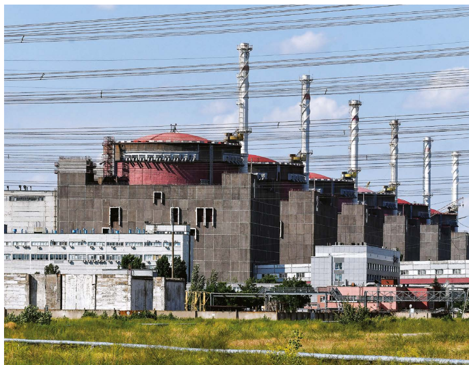
The Zaporizhzhia nuclear power plant in Ukraine, the largest in Europe.
