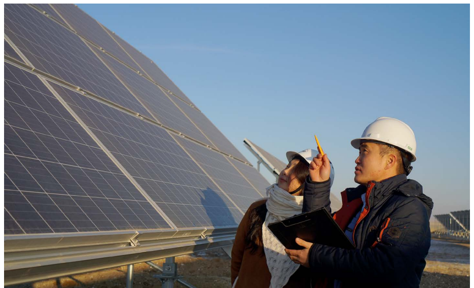
Figure 1 | Panel inspection at the Sumber Solar Plant in Mongolia. The construction of this solar plant was supported by the Green Climate Fund, the largest international fund for financing efforts to tackle global warming. However, a heavy reliance on such support is sometimes seen by poor countries as an infringement of their national sovereignty. Bauer et al. 1 report an analysis of climate policies that suggests a way to reduce the need for financial support.
