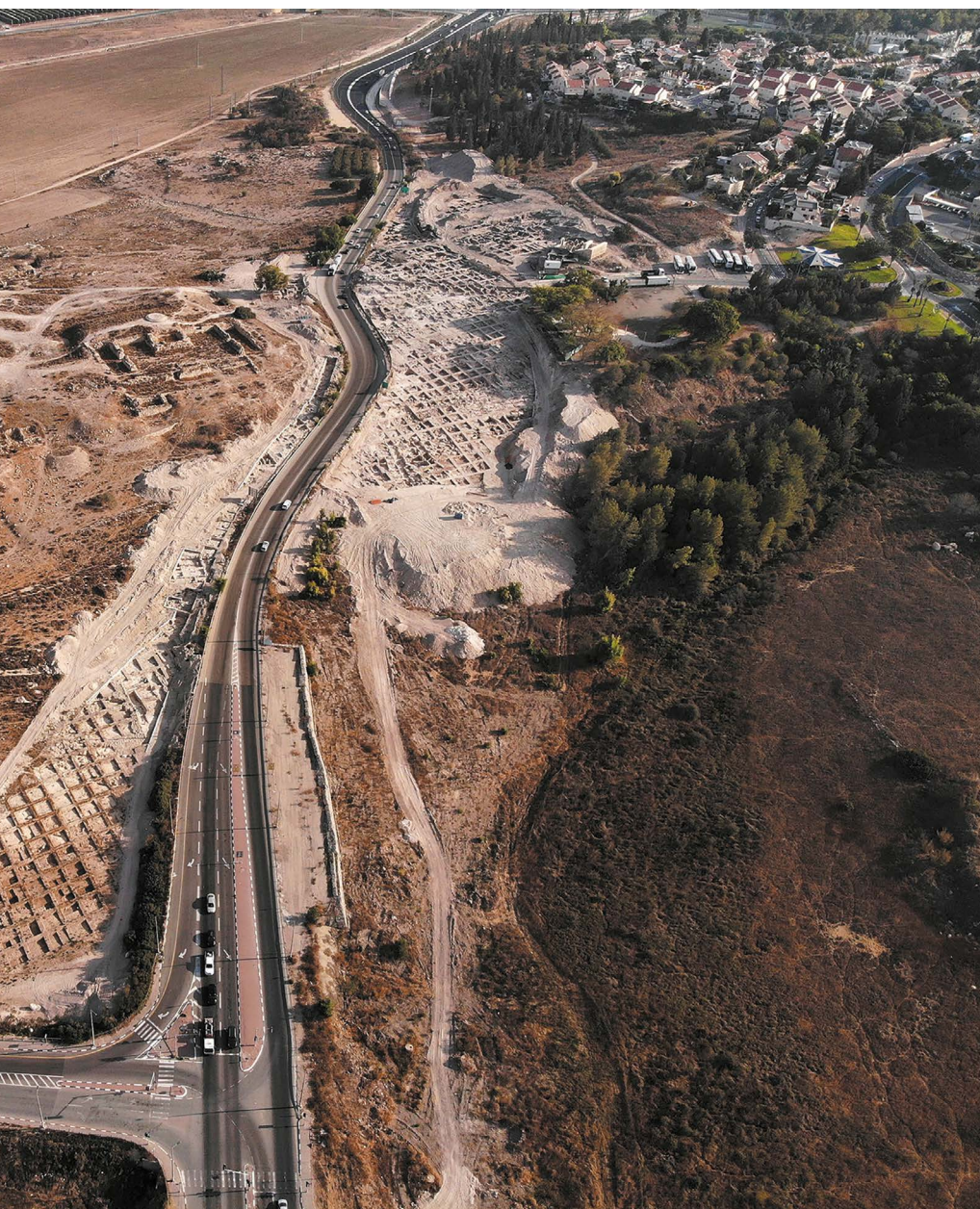
Road building threatens the site of Tel Beit Shemesh, dating to at least the seventh century BC.
