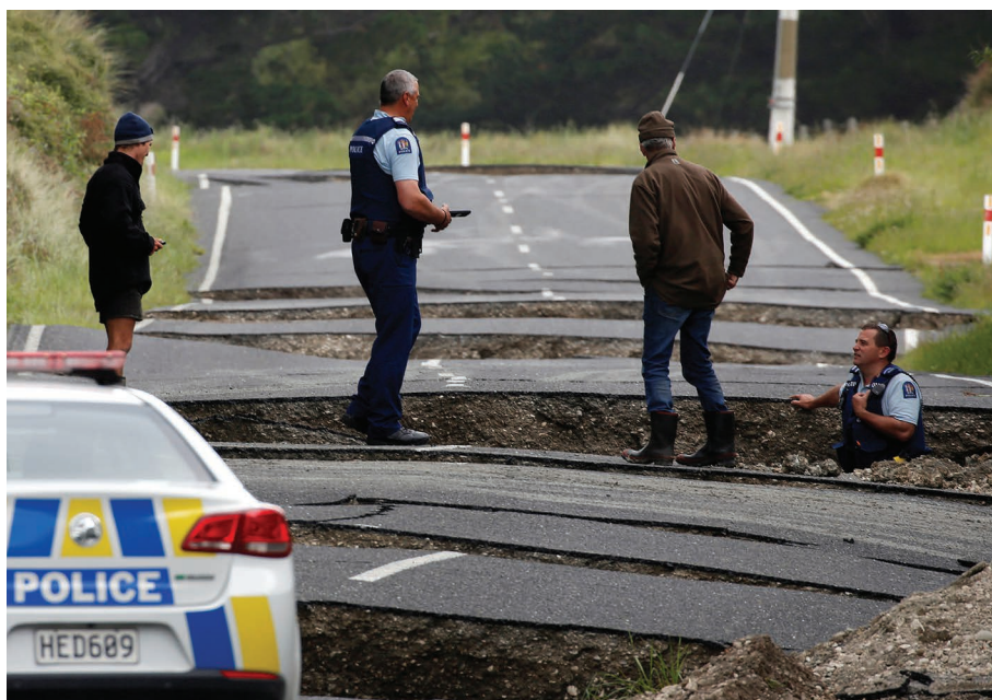
The Kaikoura earthquake in 2016 caused extensive damage on New Zealand's South Island.
