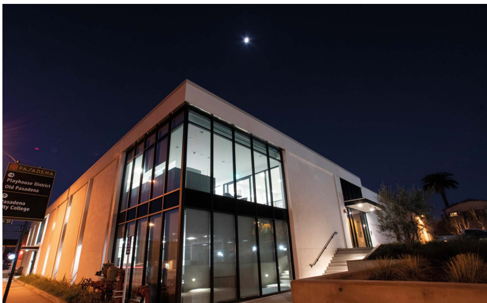
Figure 3. Expanding CSL Behring's R&D facility in Pasadena, California, US, enables the focus on cell and gene therapy that promises to advance new capabilities in this scientific platform.
