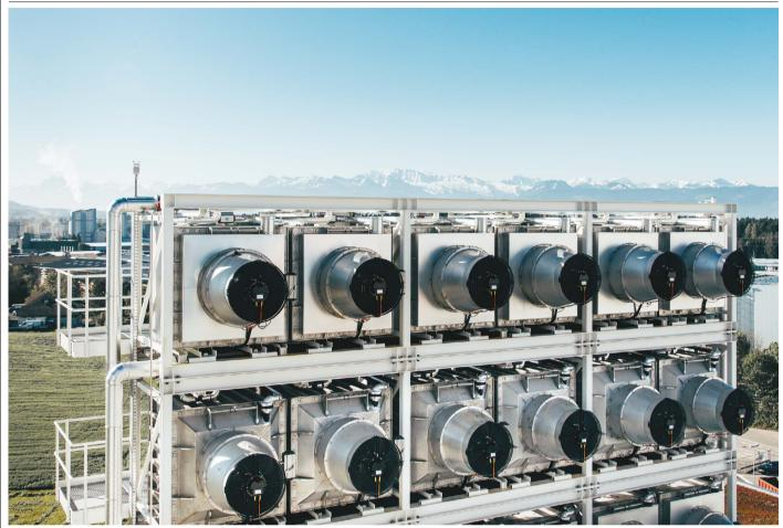
Climeworks' plant for direct air capture in Iceland removes carbon dioxide permanently from the atmosphere.
