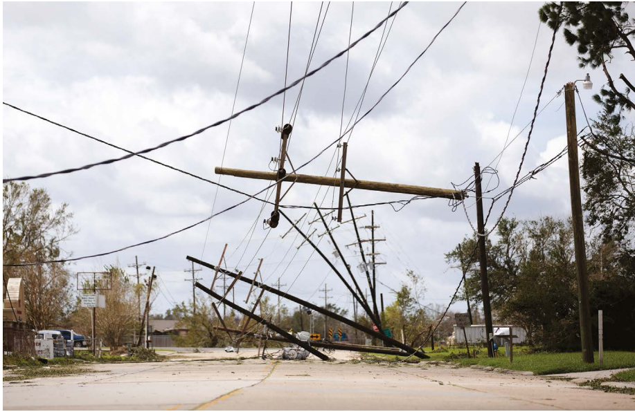
Hurricane Ida destroyed almost 30,000 utility poles in Louisiana.
