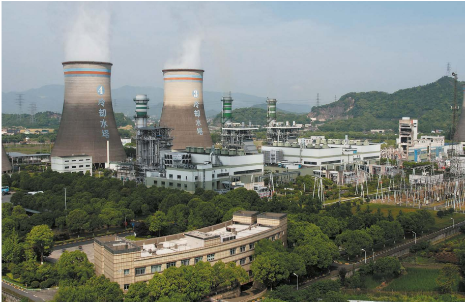
A coal-fired power plant in Hangzhou in China's Zhejiang province.
